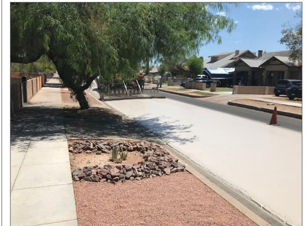
Cool pavement is a water-based asphalt treatment that is applied on top of the existing asphalt pavement.
