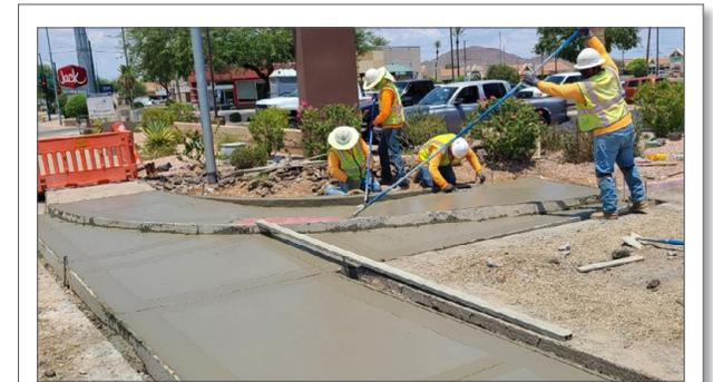
Crews install curb ramps to provide a safe route that people with disabilities can use to transition from a curbed sidewalk to roadway and vice versa.
