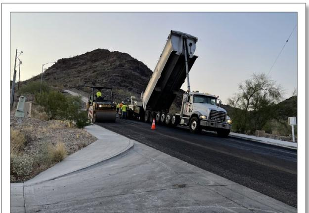
Dunlap Avenue between 7th Street and 15th Street received mill and overlay work, which includes removal of the top layer of a street (milling) followed by laying new asphalt (overlying).
